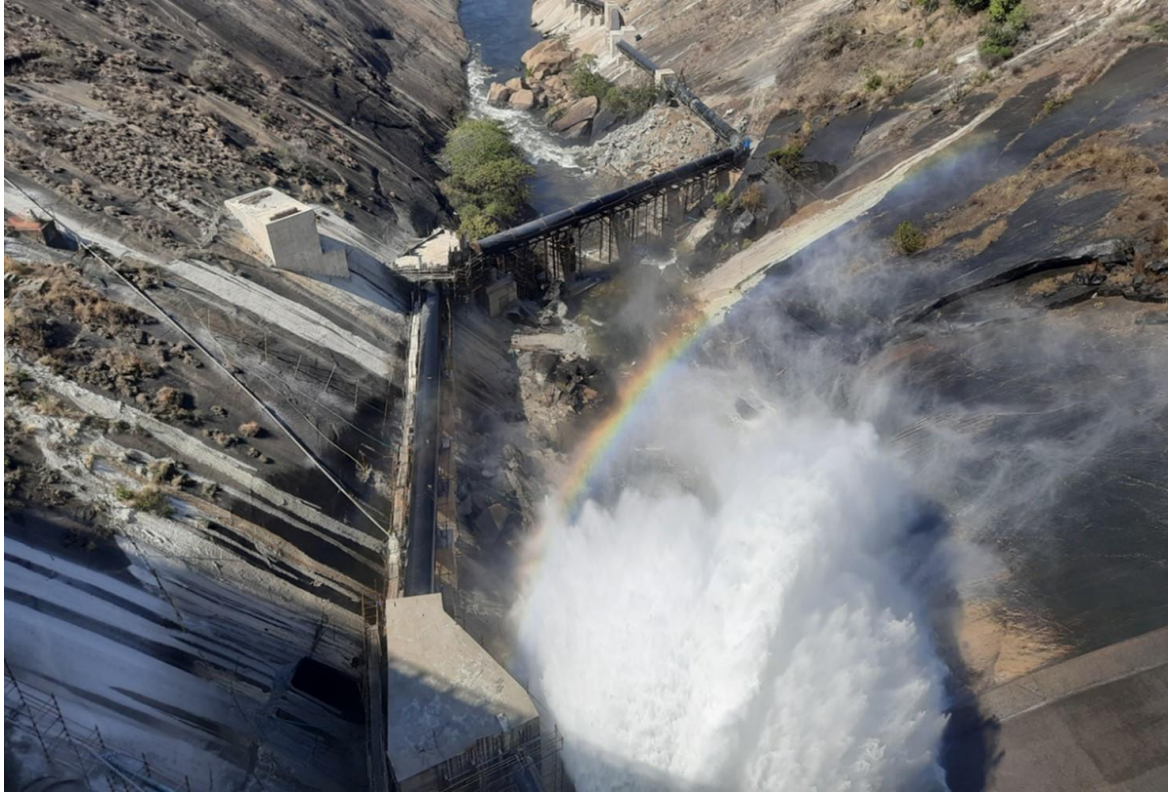
Great Zimbabwe Hydro Power Energy Project in Zimbabwe. Frontier II
